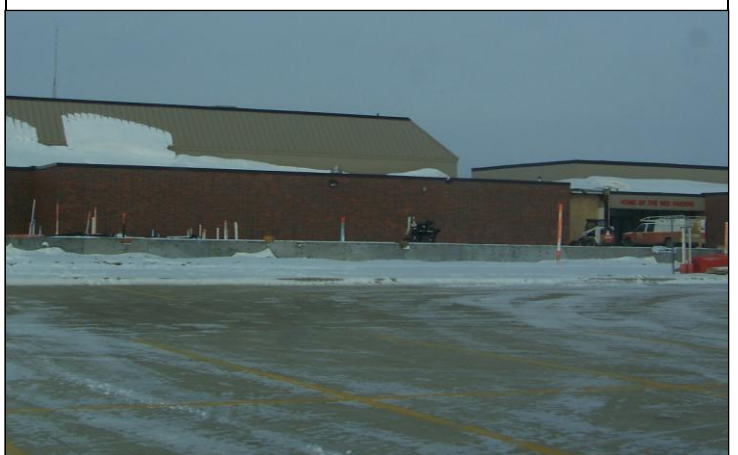
New kitchen/dining room project on east side
